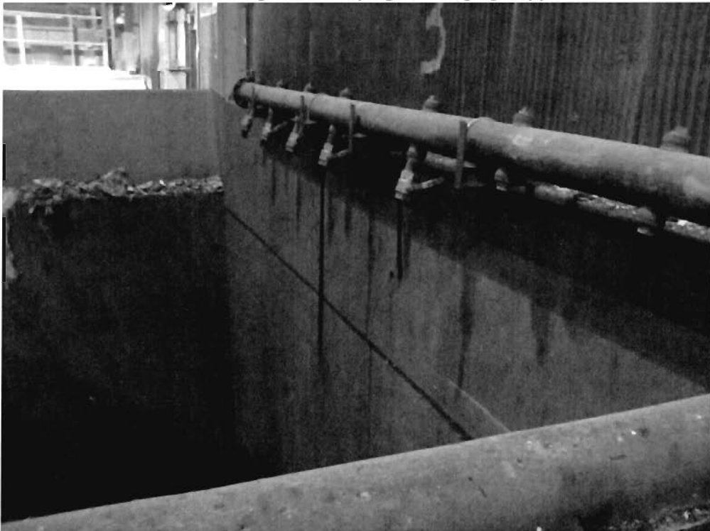
Figure 17 – Biosolids Discharging from Distribution Header to Charging Hopper
