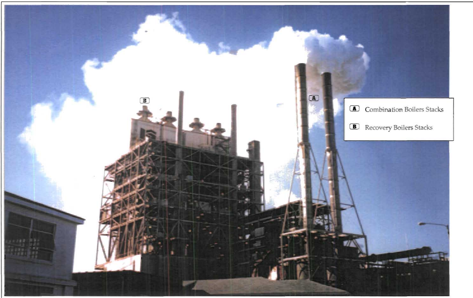
Figure 2-4. Photo of Recovery Boilers Building at SCC, Panama City
