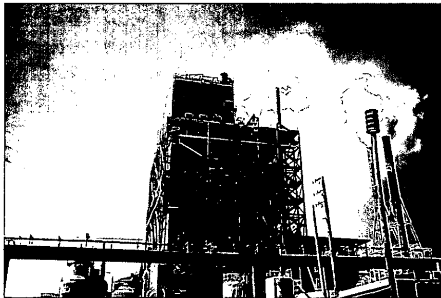
Photo 2. View From Northeast to Southwest.
