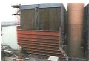
End elevation of ESP with plenum.
