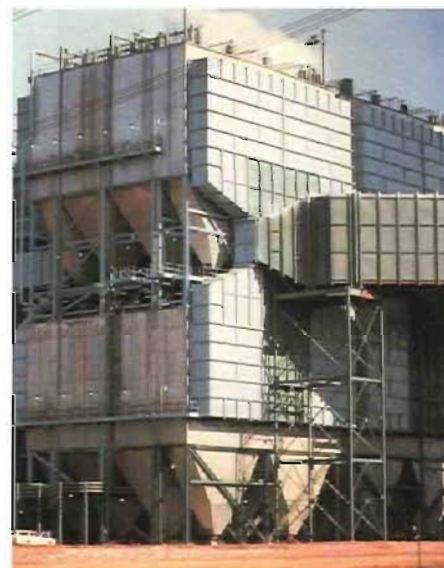
Three precipitators on pulverized coal boilers — Dutch Gap, Virginia.
