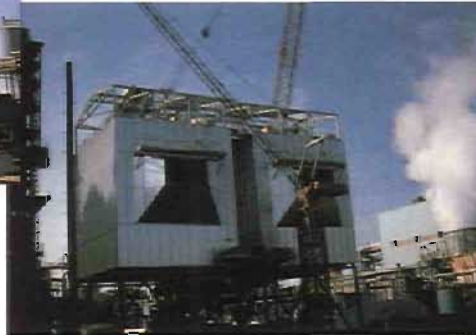
◀ ESP's in position prior to roll-in.
