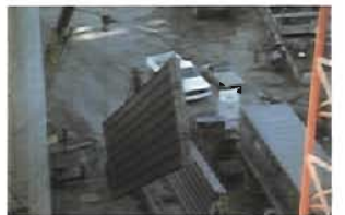
Modulok collecting plates being lifted off truck.
