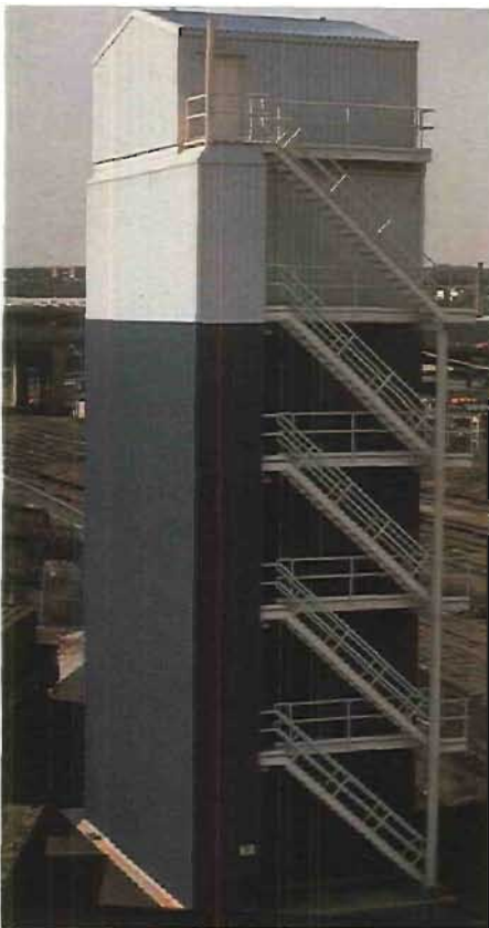
Second generation test tower for life testing of precipitator components.
