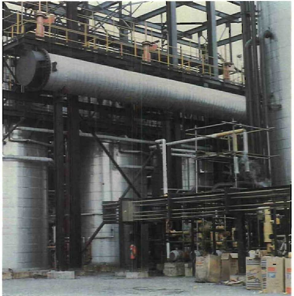
Three 130 tube gas detarrer precipitators — East Chicago, Illinois.
