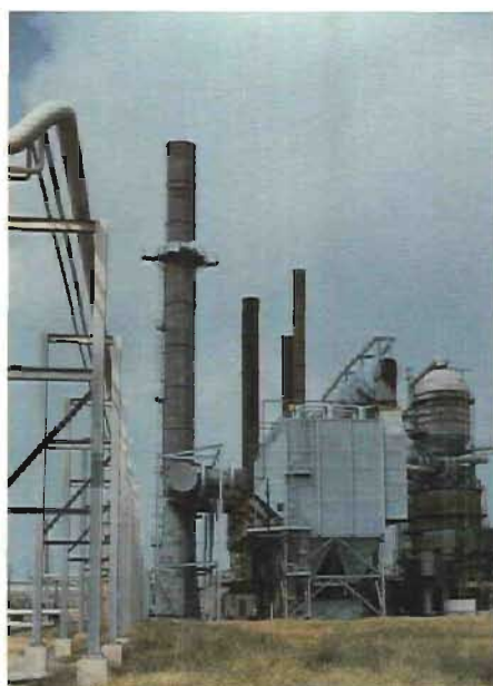
Four 211,300 ACFM fluid catalytic precipitators — Texas City, Texas.
