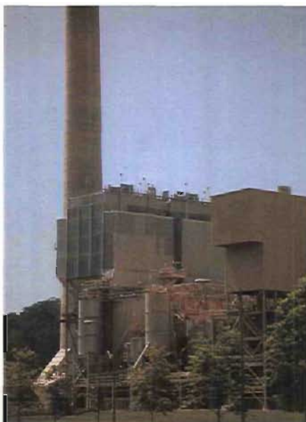
Two precipitators on two process rotary kilns — Festus, Missouri.
