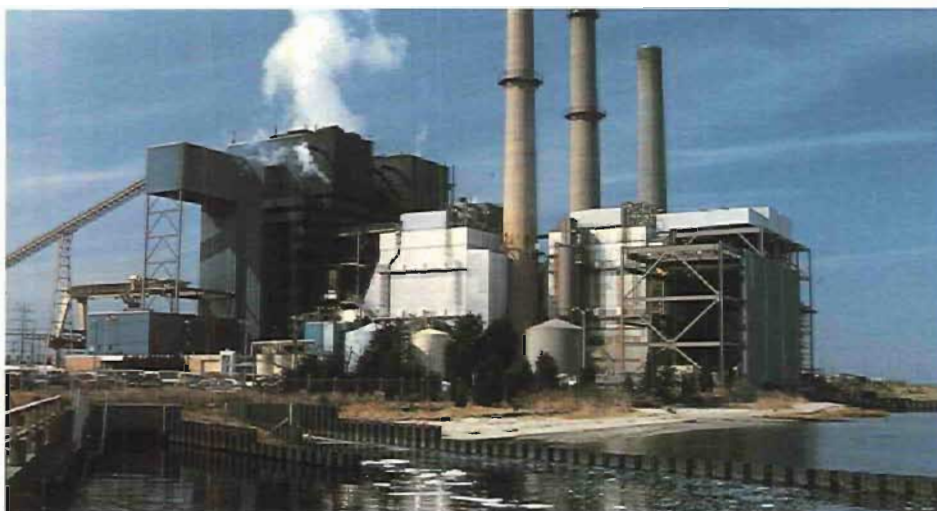
Two Rigitrode precipitators on cyclone boilers — Beesley's Point, New Jersey.
