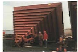
Preassembled hopper waiting transport to erection site.
