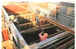
Collecting plates being moved into position.
