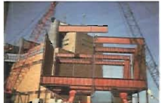
Erection of ESP casing and roof girders.
