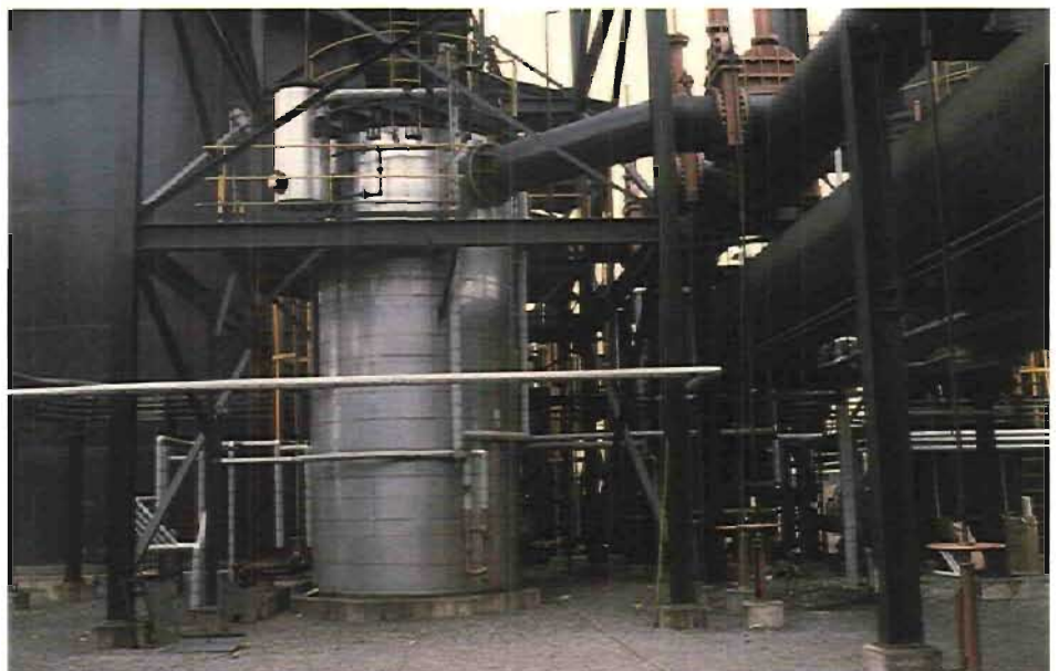
One 89 tube fuel gass detarrer — East Chicago, Illinois.
