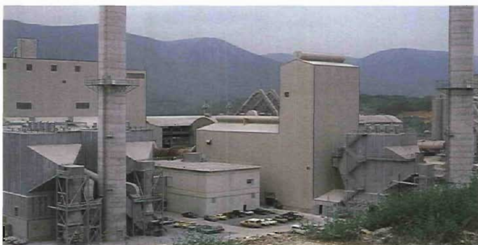
Two precipitators on two roller mills (left) and one precipitator on traveling grate preheater kiln (right) — Roanoke, Virginia.
