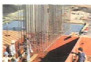
Rigirode frame being positioned between collecting plates.
