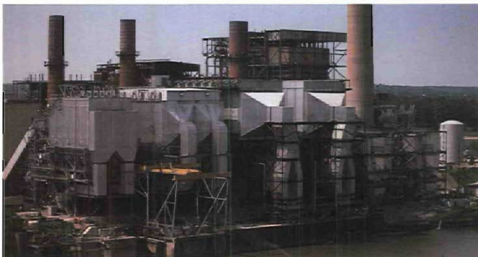
Three precipitators on pulverized coal boilers — Dutch Gap, Virginia.
