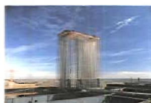
Rigirode bus section being lowered into the ESP casing.
