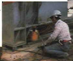
► Hydraulic jack used to lift ESP for roller insertion.
