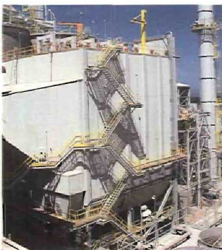
Two precipitators on two process rotary kilns — Festus, Missouri.
