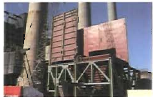
Erection of ESP casing side panels.
