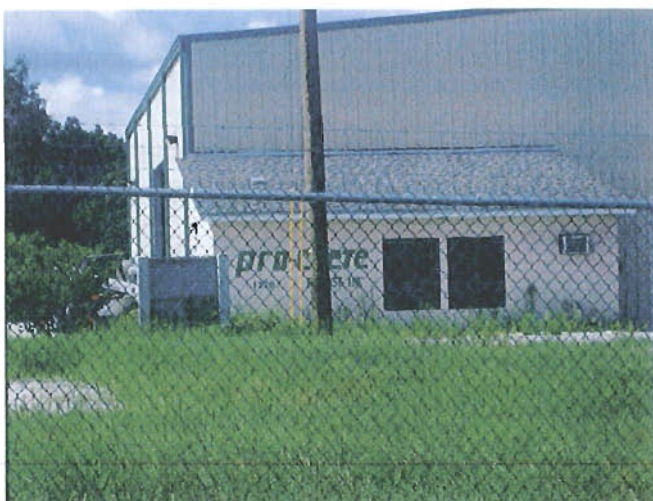
Photo ID No.3 7/14/11 11AM Close-up of main building and fence.
