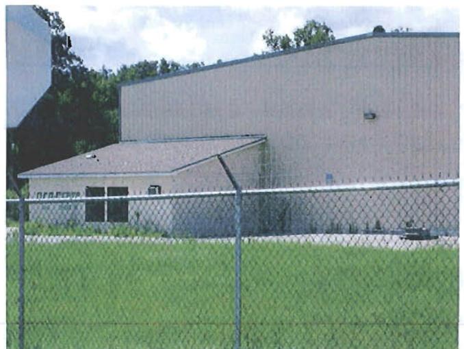
Photo ID No.4 7/14/11 11AM Main building from second entrance.
