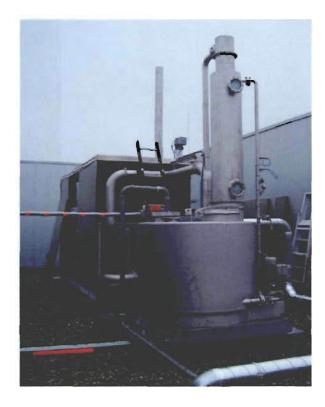
The first step is the EO Balancer, where water is circulated from a buffer tank over a column, to generally equalize the variation in the incoming concentration of EO; such that when levels of incoming EO are high, the system absorbs EO in the water and when levels of incoming gas are low the system strips EO out from the water.
