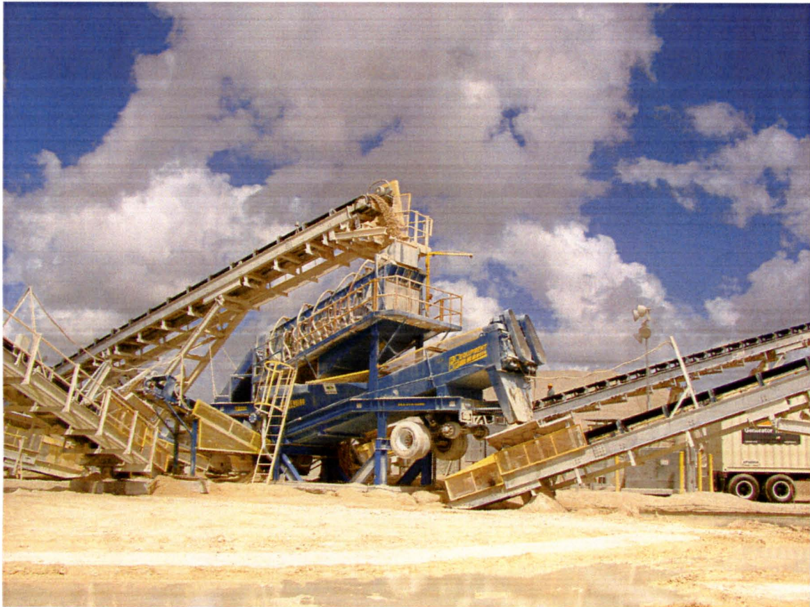
Conveyor Discharge into Wet Screen
