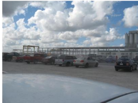
Picture ID No. 003 South-west photo of parking lot after wind.
