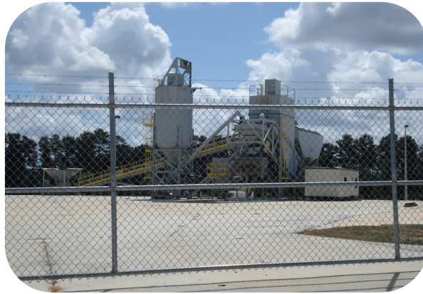
Shows concrete batching operation
