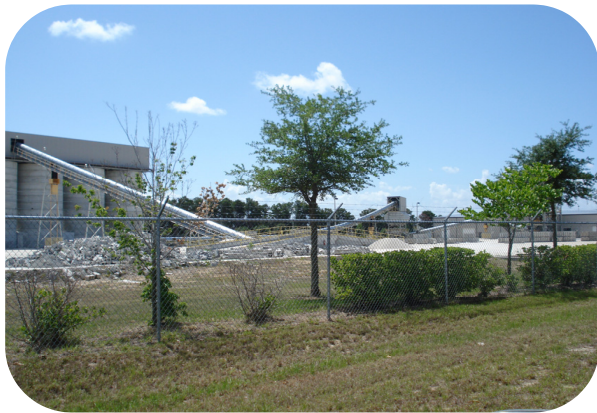
Shows that there is concrete piles
