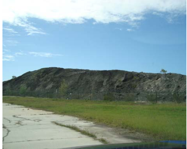
Stock pile of soil/asphalt located adjacent to the facility.
