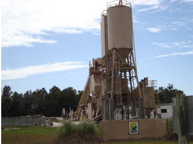
EU001 – Cement and fly ash silos.
