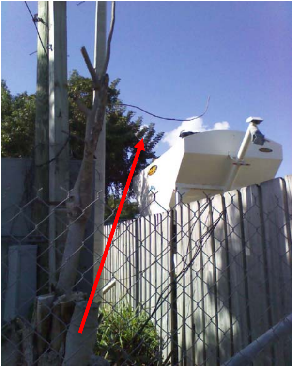
Inspection hatch location, on top
