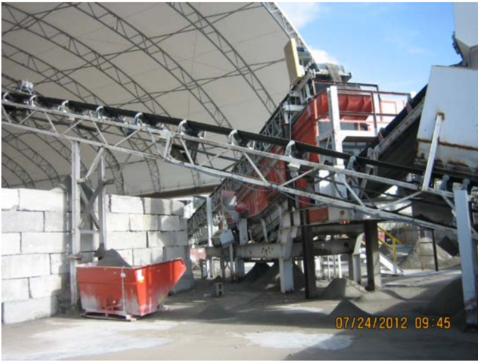
Photo ID No: IMG_467 – Pile Conveyor No. 3 with Screen No. 2 in background.
