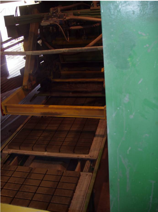
Photo ID No: 1050372_Photo_01_24_2012-31 Time: Approx. 12:30 PM Inside of Plant 1, view of paver molding and manufacturing. Camera is facing approx. SE.
