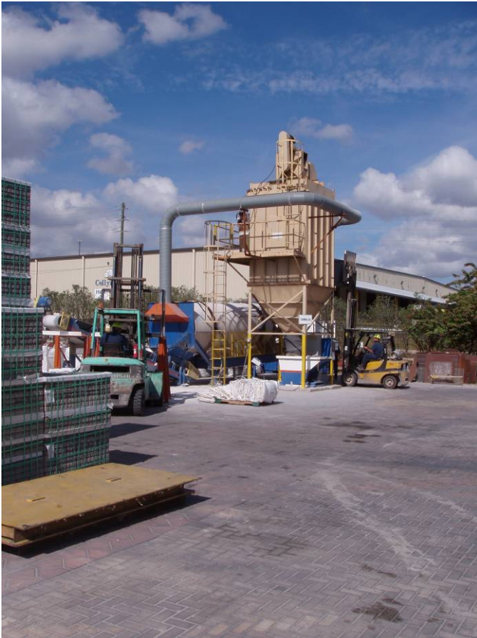
Photo ID No: 1050372_Photo_01_24_2012-13 Time: Approx. 12:20 PM Paver tumbler machine with central dust collector (EU014) just West of Plant 1. The camera is facing approx. NE. This photograph shows the approximate perspective from where the VE test was conducted for the paver tumbler machine with central dust collector (EU014). In this photograph, the operator on the yellow-colored fork-lift delivers loads of pavers into the tumbler, which is the horizontal cylinder that is white in color. The South face of the tumbler is blue with an orange ventilation system that receives dust from the tumbler. The dust flows through the grey ducts up to the central dust collector (unit that is light-yellow or beige in color). The dust then collects at the base of the central dust collector in a storage bin that is white and blue in color with an orange stripe in the center. The operator on the mint-green-colored fork-lift removes filled bags of pavers from the paver loading area.
