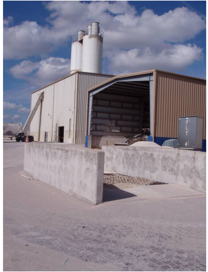
Photo ID No: 1050372_Photo_01_24_2012-12 Time: Approx. 11:45 AM Underground drop-off pit with grates for aggregates, outside of Plant 4, to be delivered to storage bins by conveyor belt. Camera facing approx. NE. In the background, Plant 1 and the sand hanger are visible.
