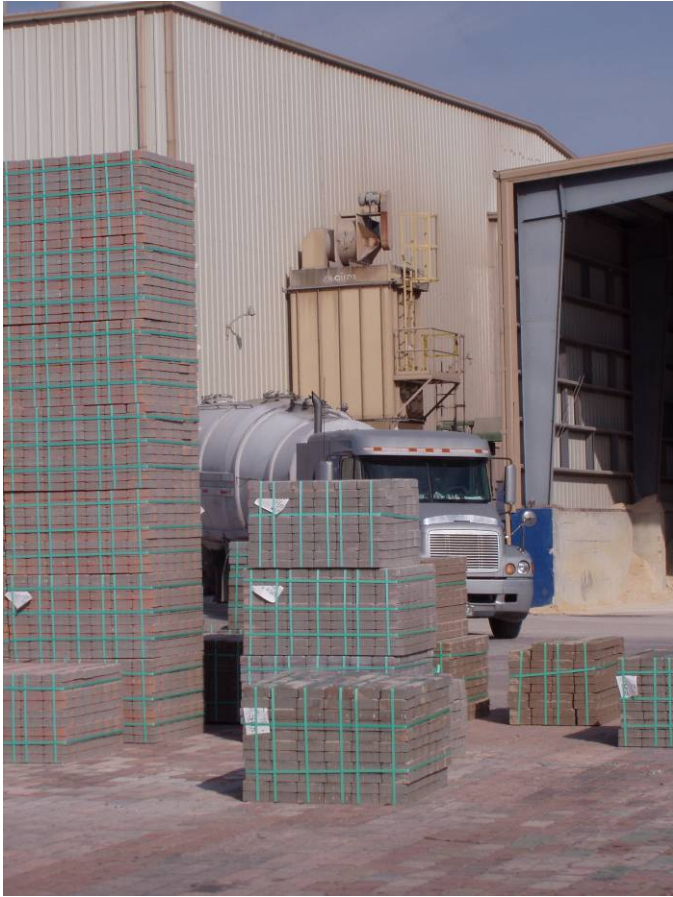
Photo ID No: 1050372_Photo_01_24_2012-6 Time: Approx. 10:30 AM. Photo of the Plant 1 central dust collector (EU004), which is directly behind the truck. Camera facing approx. NW. The central dust collector picks up dust from two mixers (for batching) in Plant 1 and collects dust in a bin.
