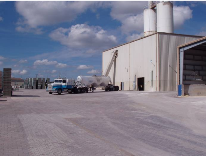
Photo ID No: 1050372_Photo_01_24_2012-9 Time: Approx. 11:45 AM Grey cement truck finishing the filling of the Plant 1 grey cement silo (EU001) after the second VE test had been conducted at Hanson Hardscape Products Facility on 01/24/2012. Camera facing approx. WNW.
