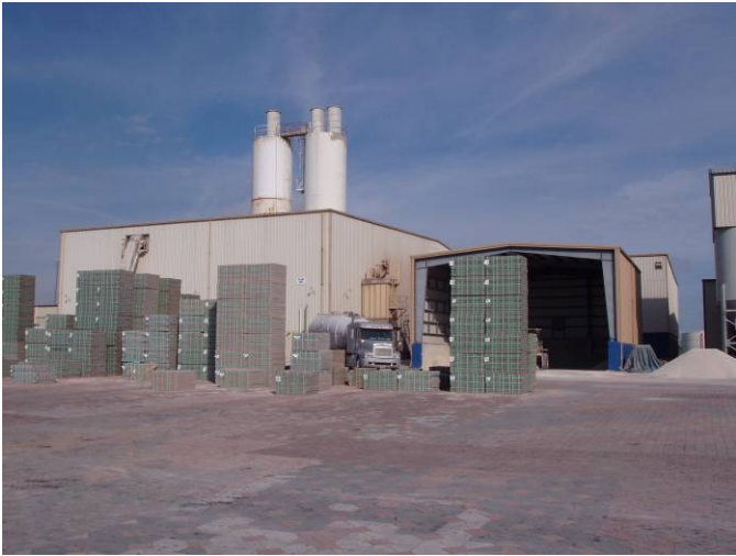
Photo ID No: 1050372_Photo_01_24_2012-3 Time: Approx. 10:30 AM. View of Plant 1, camera facing approx. NNW. This photograph shows the approximate perspective from where the VE tests were conducted for the Plant 1 silos (EU001, EU002, and EU003) and the Plant 1 central dust collector (EU004). The two silos are, from left to right, grey cement silo (EU001) and a split silo for white cement (West portion, EU002) and for cement supplement, or slag (East portion, EU003). The Plant 1 central dust collector (EU004) is the light-yellow-colored structure in between Plant 1 and the sand hanger (building with open face). The central dust collector is directly behind the truck, which was filling the cement supplement silo.
