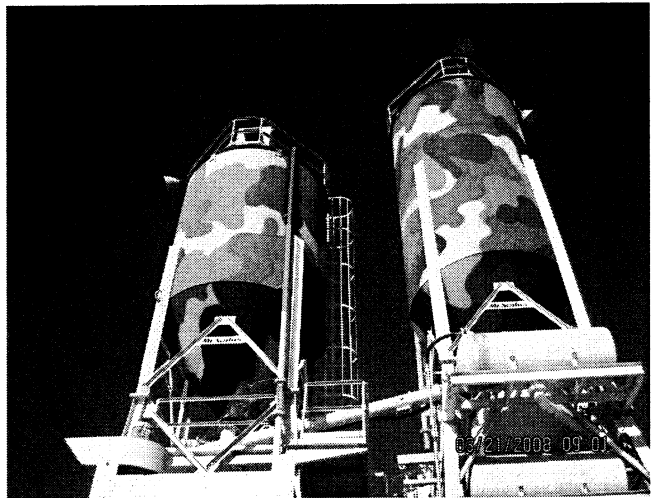
Photo ID No. / Date / Time: Inland Mat 032108 (2) Cement and flyash silos / 3/21/08 / 10:01
