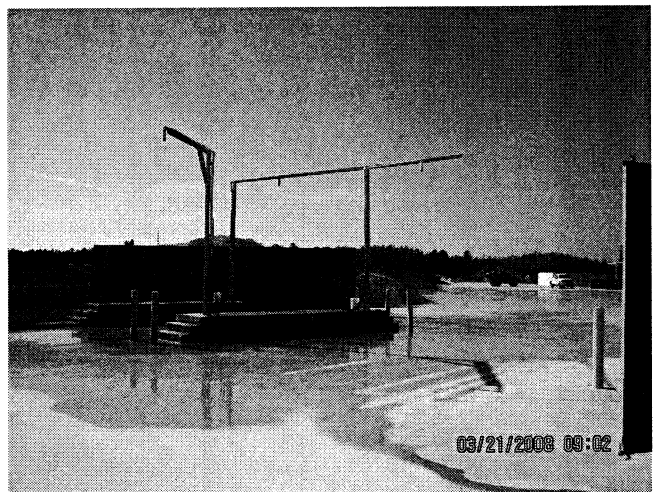
Photo ID No. / Date / Time: Inland Mat 032108 (4) Stock piles / 3/21/08 / 10:02
