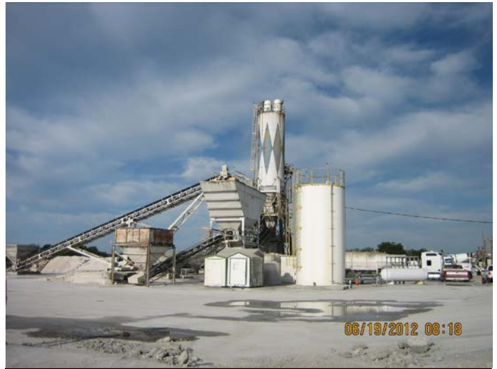
Photo ID No: IMG_488 – 2 silo top dust collector exhaust points are visible from this location ( Emission Unit Nos. 002 and 003).
