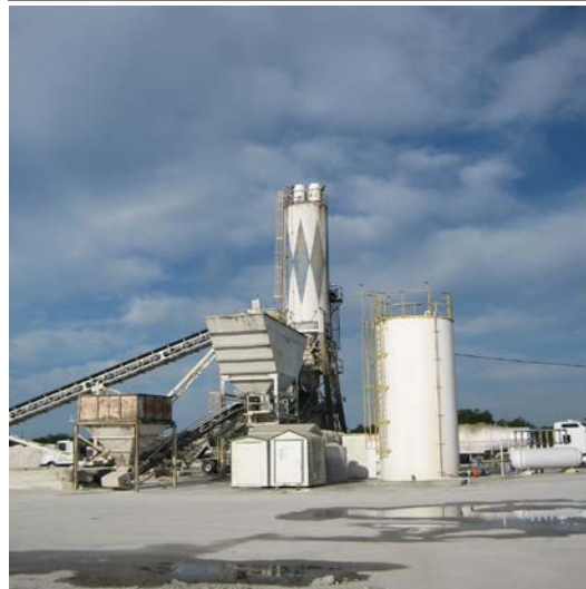
Photo ID No: IMG_488 – 2 silo top dust collector exhaust points are visible from this location ( Emission Unit Nos. 002 and 003).
