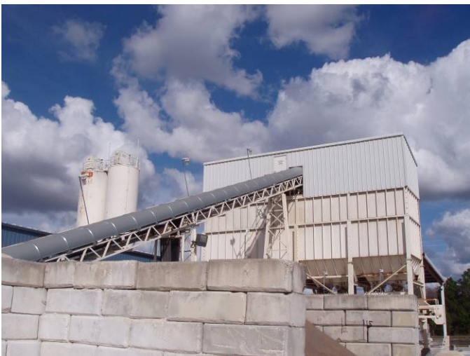
Photo ID No: 1050350_Photo_01_24_2012-8 Time: Approx 14:00 PM View of silos from approximate perspective of where VE tests were conducted for EU005 and EU006; camera facing approx. ENE.
