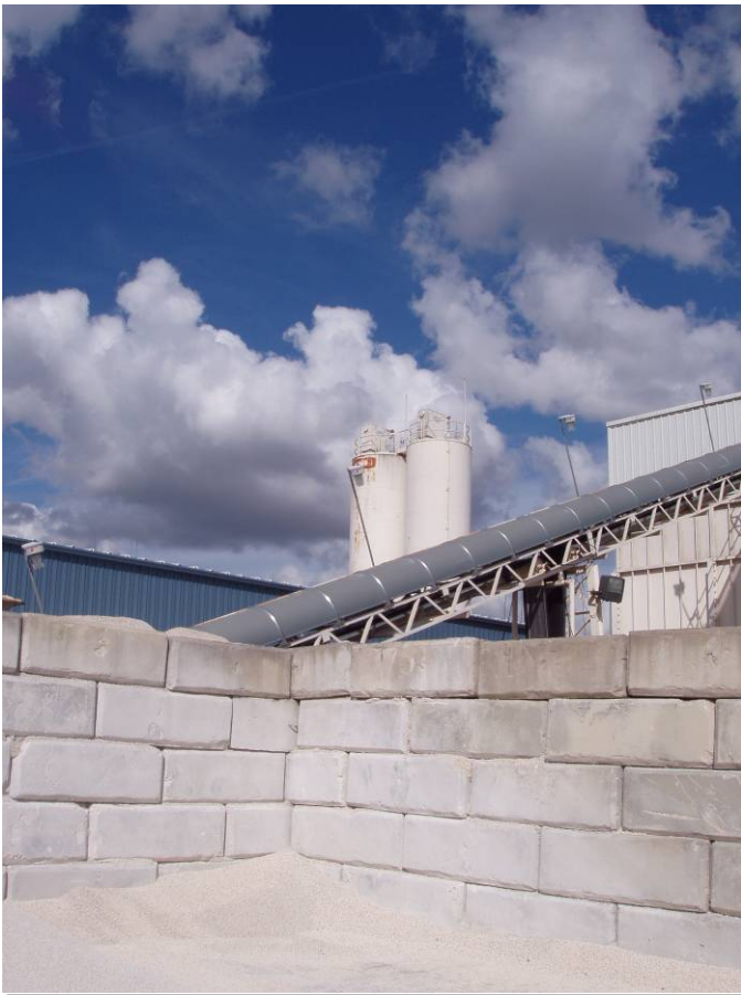
Photo ID No: 1050350_Photo_01_24_2012-7 Time: Approx 14:00 PM Approximate view from where VE tests were conducted for EU005 and EU006; camera facing approx. NE.
