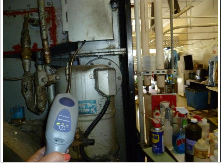
**Description:** [The halogen detector leak detector sounded alarm when at rear of dry to dry near right side of lint trap near valve.]
