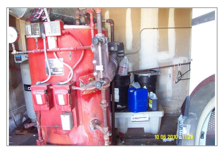
Project Id:75677Permit No: 1030324-004-AGInspector:Shea JacksonInspection Date : 10/6/2010Source (EU):New, Small Perchloroethylene Dry Cleaner: One Dry-to-dry machine (2001),<br/>Frigo -Sec Model M280-35, serial # 103L9060 with a refrigerated condenser.1<br/>exempt 25 hp natural gas fired boiler is on-site.
