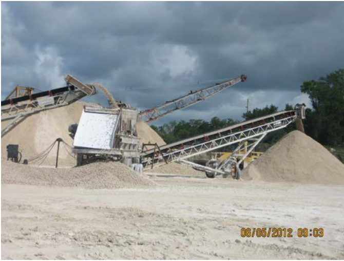
Photo ID No: IMG_428 – Power Screen Unit. Facility ID No. 7775703.
