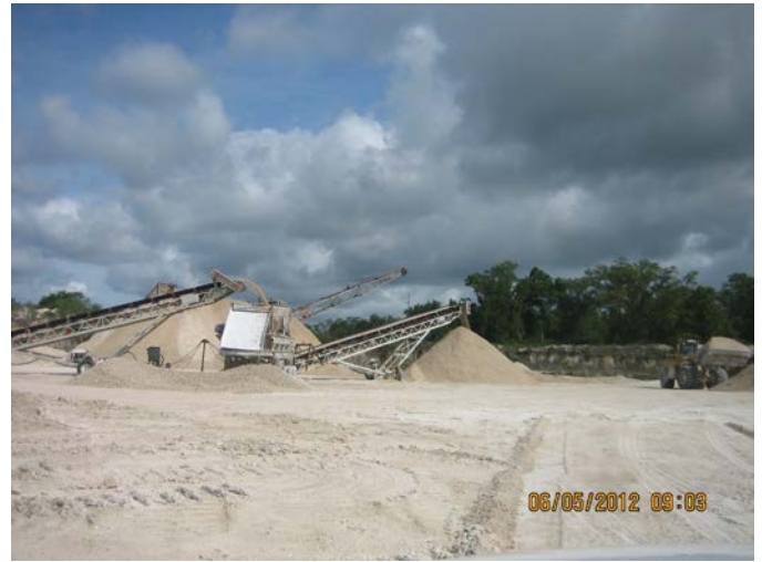
Photo ID No: IMG_425 – Screen Facility ID No. 7775703
