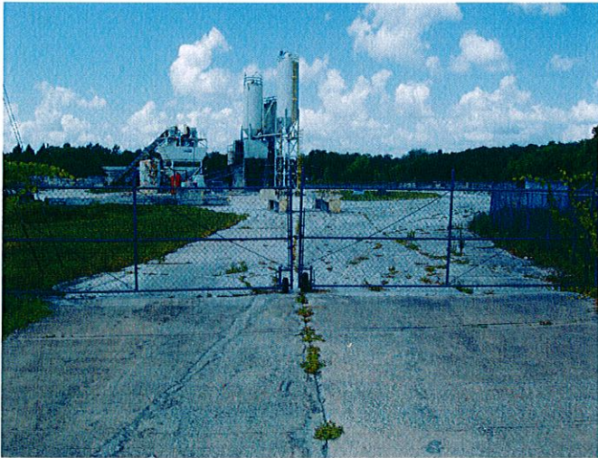
Photo ID No. / Date / Time: Picture 001 05-26-2011 11:15 Entrance to Inactive facility.
