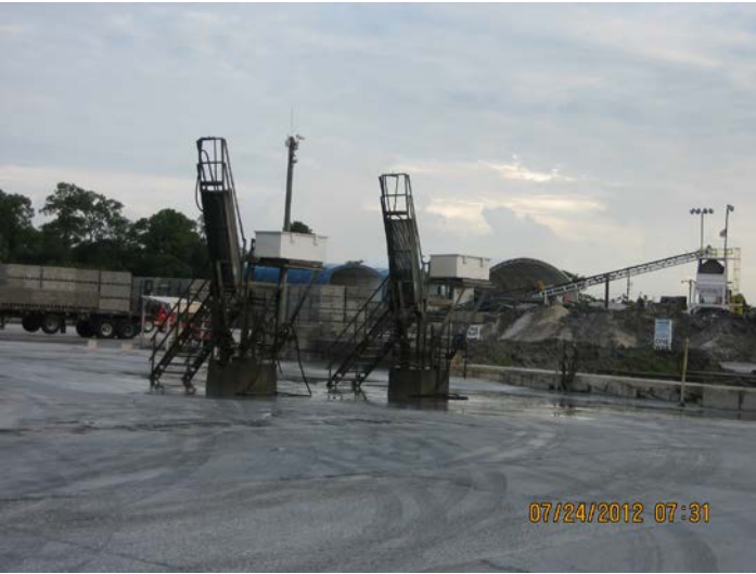
Photo ID No: IMG _436 – This photo shows adequate wetting of roadways/yard.
