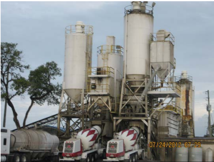
Photo ID No: IMG_432 – Loading 2 cement trucks and silo simultaneously.
