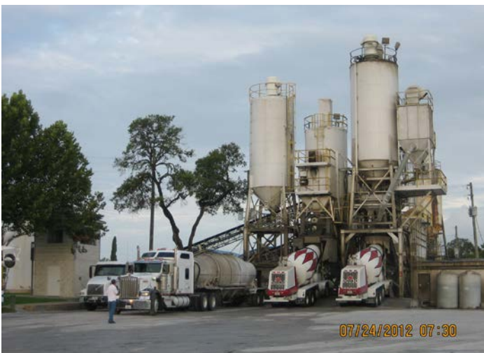
Photo ID No: IMG_433 – Arrival of second truck for silo loading.
