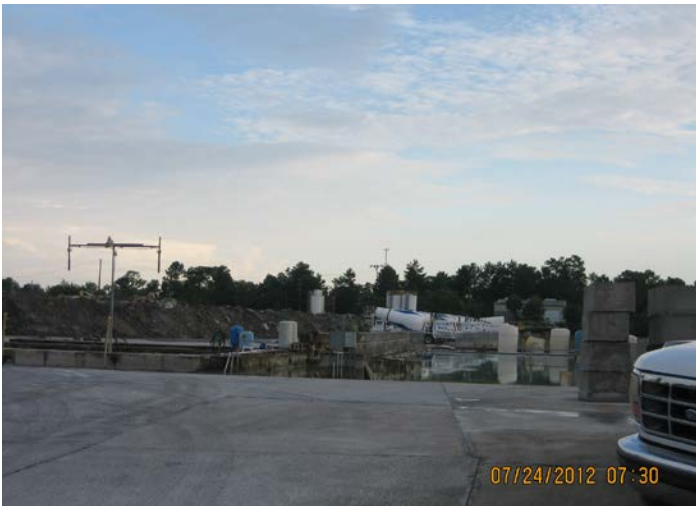
Photo ID No: IMG_434 – This photo shows view of paved roadway.
