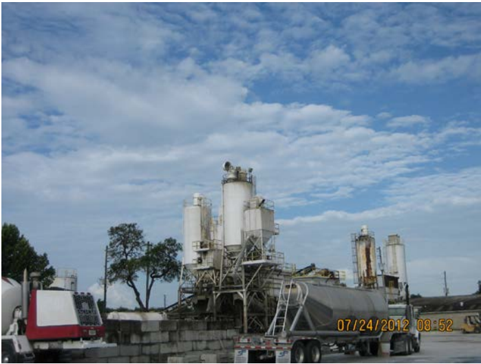
Photo ID No: IMG_452 – This photo shows a wide view of plant and a B. E. T. ER Mix employee inspecting EU11 dust collector.
