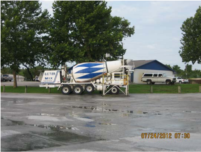
Photo ID No: IMG _435 – This photo shows adequate wetting of roadways/yard.
