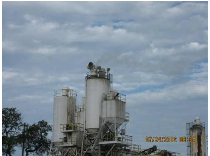
Photo ID No: IMG_448 – This photo shows a slightly zoomed view of flyash release from new dust collector for Emission Unit No. 11 and shows how quickly release began tapering off.
