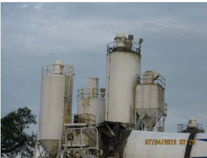
Photo ID No: IMG_431 – 6 Dust Collector exhaust points are visible from this location.
