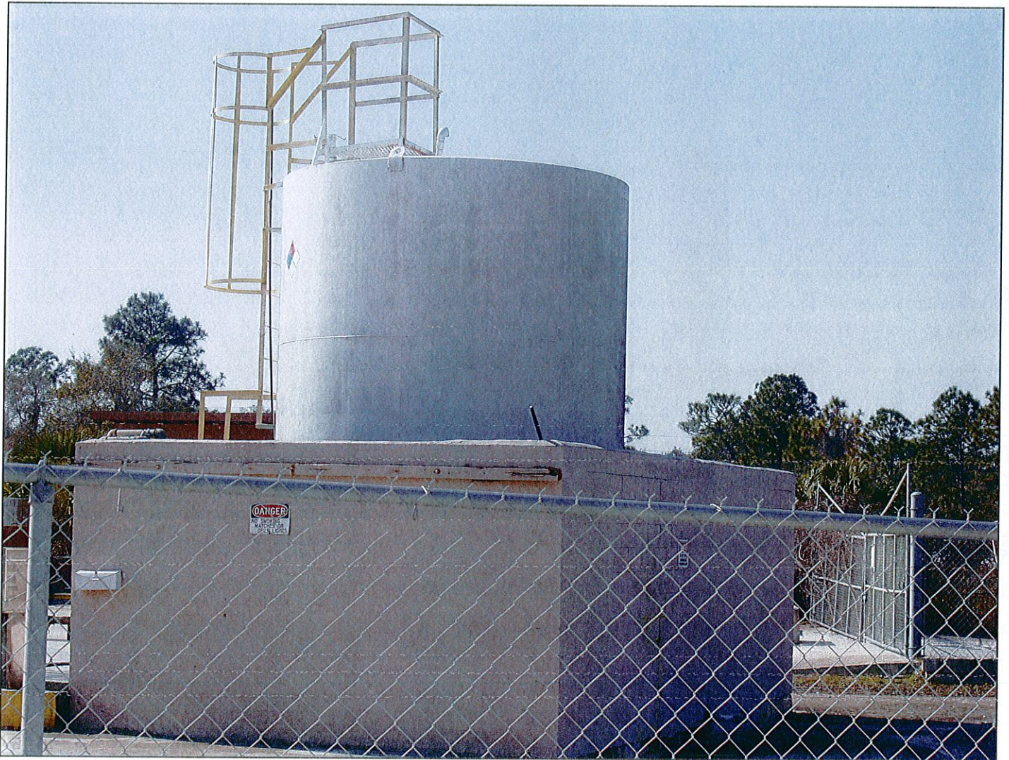
Photo ID No. / Date / Time: IMG_0962 / 02-16-2011 / 1100 Closed Facility
