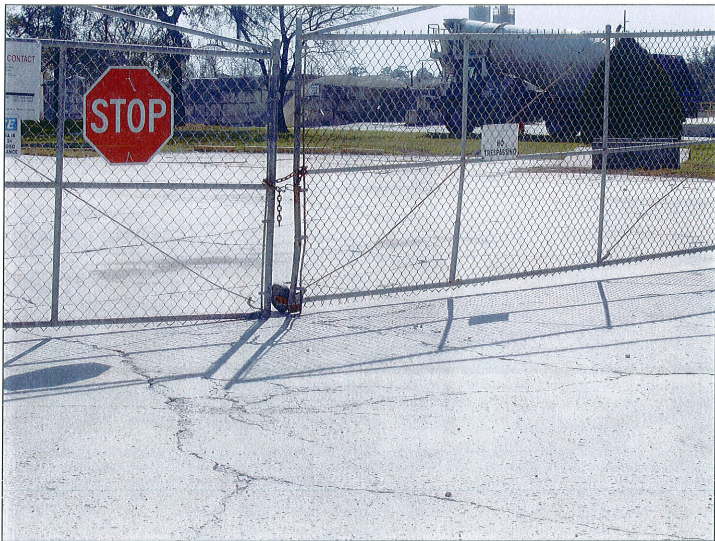
Photo ID No. / Date / Time: IMG_0962 / 02-16-2011 / 1100 Locked Gate at Facility
