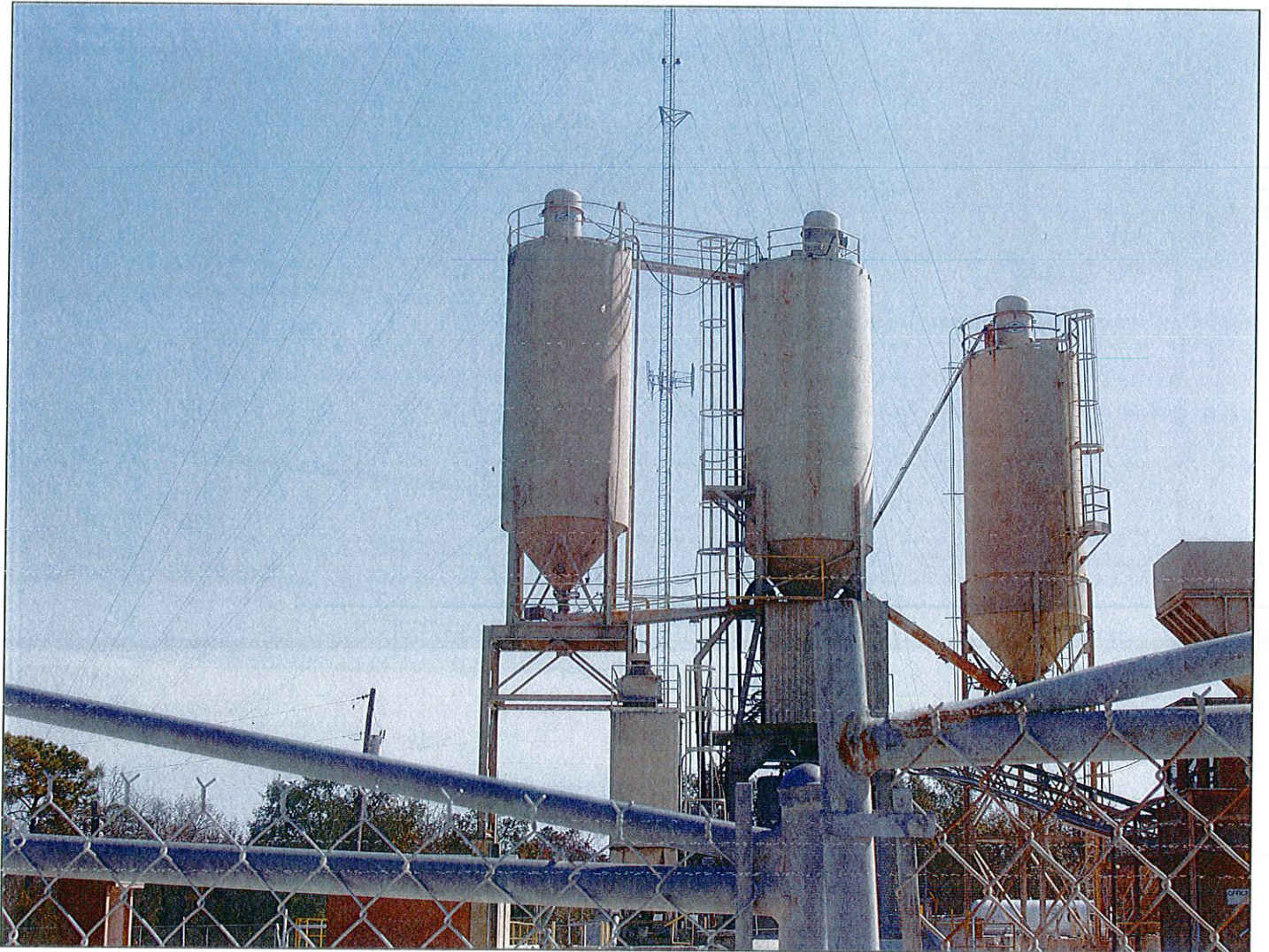
Photo ID No. / Date / Time: IMG_0962 / 02/16/2011 / 1100 Three Storage Silos at Closed Facility
