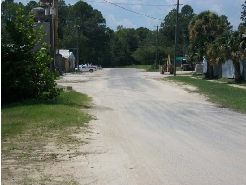
View from East of Jerkins Concrete Batch Plant. Entrance and exit to the plant is on left side of picture.
