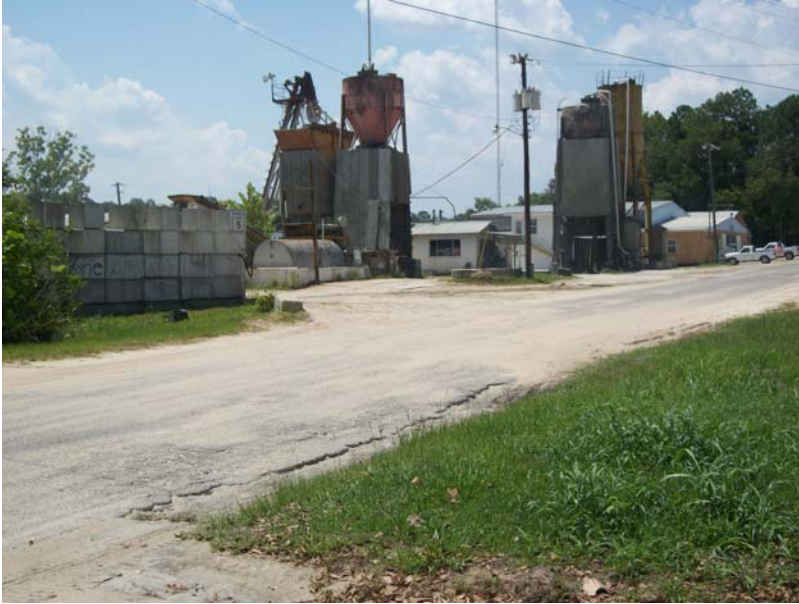
View from Southeast of Jerkins Concrete Batch Plant across West Pennsylvania Avenue.
