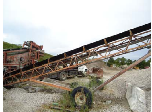
Existing stationery crusher unit showing convey belt (7775112).
