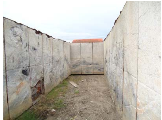
Inside of ACI unit with dirt floor.
