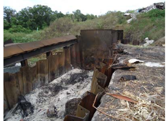
Existing in-ground ACI showing waste burn material/ash (1270154).
