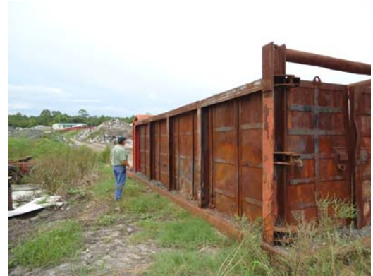
Outside of ACI unit.
