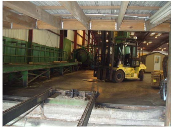
Photo ID No: 1190048_Photo_03_01_2012-007 Time: Approx. 10:00 AM Forklift and other equipment for loading wood products onto horizontal cylinder for CCA treatment. The forklift is on a pad with borders to help prevent any possible leaks from spreading to the rest of the building or environment. The camera is facing approx. N.
