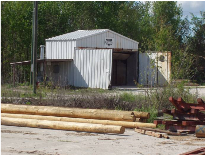
Photo ID No: 1190011_Photo_03_01_2012-016 Time: Approx. 14:45 Dry Kiln located just Northwest of Kiln 2 (EU002, southwest Kiln). The camera is facing approx.W.
