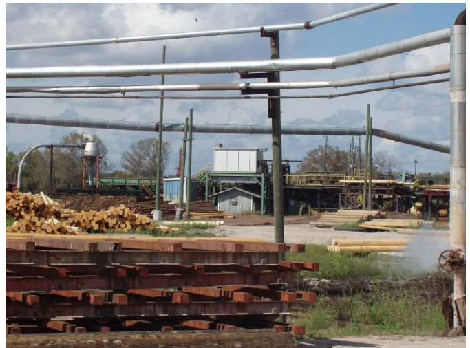
Photo ID No: 1190011_Photo_03_01_2012-014 Time: Approx. 14:30 View of pole manufacturing line in background of photo. The camera is facing approx. NW.
