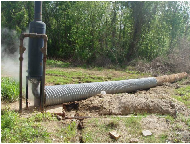
Photo ID No: 1190011_Photo_03_01_2012-011 Time: Approx. 14:15 Blowdown pipe for #####. The camera is facing approx. SW.
