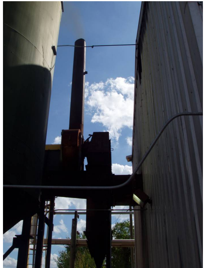
Photo ID No: 1190011_Photo_03_01_2012-005 Time: Approx. 14:00 Stack from Hurst Boiler, visible in between the sawdust storage silo and the building containing the Hurst and ABCO boilers. This stack is located on the East side of the building. Next to and below the stack is the Hurst multicyclone collector, which collects particulate matter from the exhaust of the boiler and transfers the particulate matter into a drum (as described in a diagram from air construction permit 1190011-003-AC). The camera is facing approx. S.
