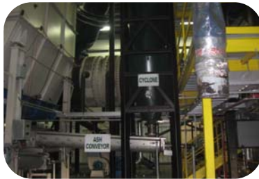
High efficiency high temperature cyclone
