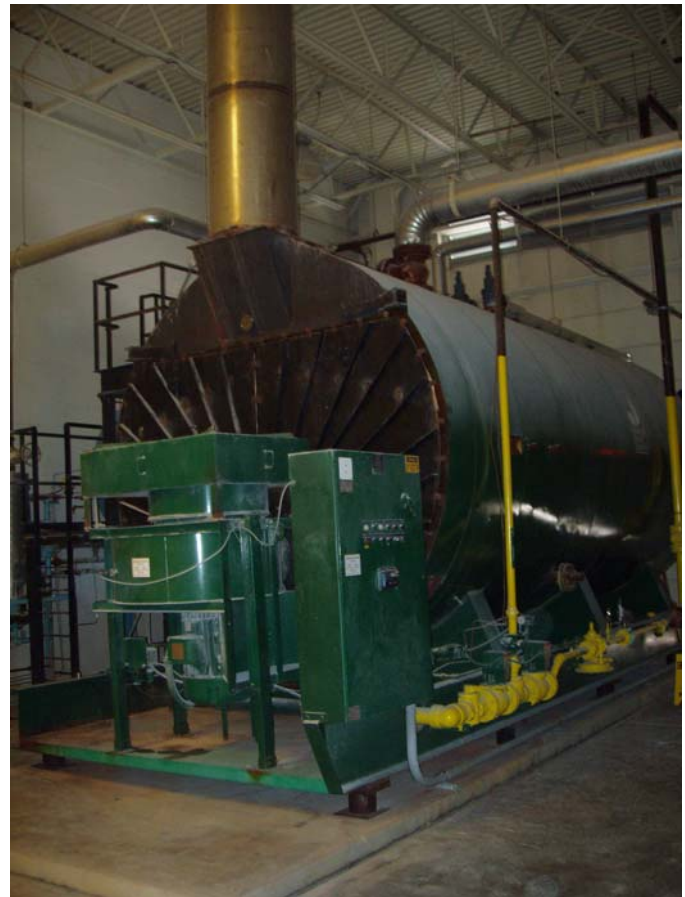
Photo ID No: 1050276_Photo_05_10_2012-013 Time: Approx. 11:30 AM Another view of the Johnston boiler, exempt from air operating permitting, which supplies steam to the autoclaves at the facility. The camera is facing approx. SE.
