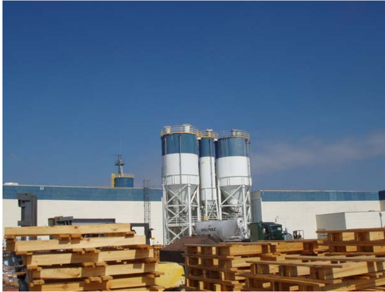
Photo ID No: 1050276_Photo_05_10_2012-002 Time: Approx. 09:45 AM Lime being loaded by truck into the North compartment of the South Lime Storage Silo (EU002-EP001). The camera is facing approx. NE.
