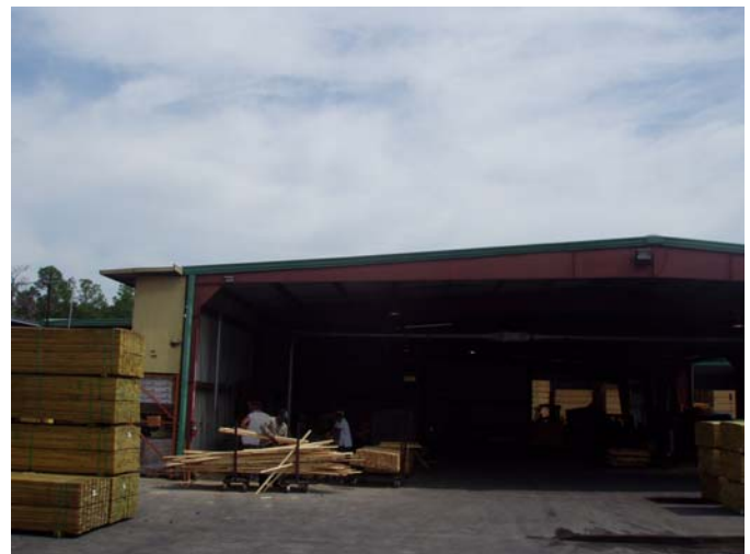
Photo ID No: 1050244_Photo_05_15_2012-006 Time: Approx. 10:45 AM West side of building containing sawing equipment. The camera is facing approx. N.
