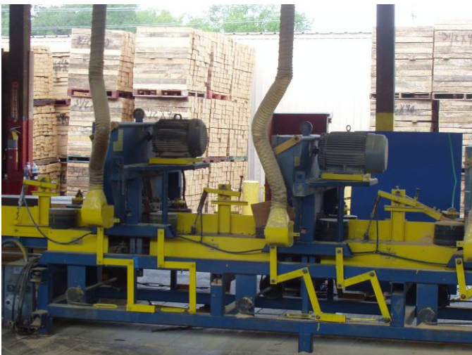
Photo ID No: 1050128_Photo_03_29_2012-004 Time: Approx. 12:00 PM Sawing equipment located inside small West cutting shed. Pickup points for dust are shown in the photo. The camera is facing approx. WSW.
