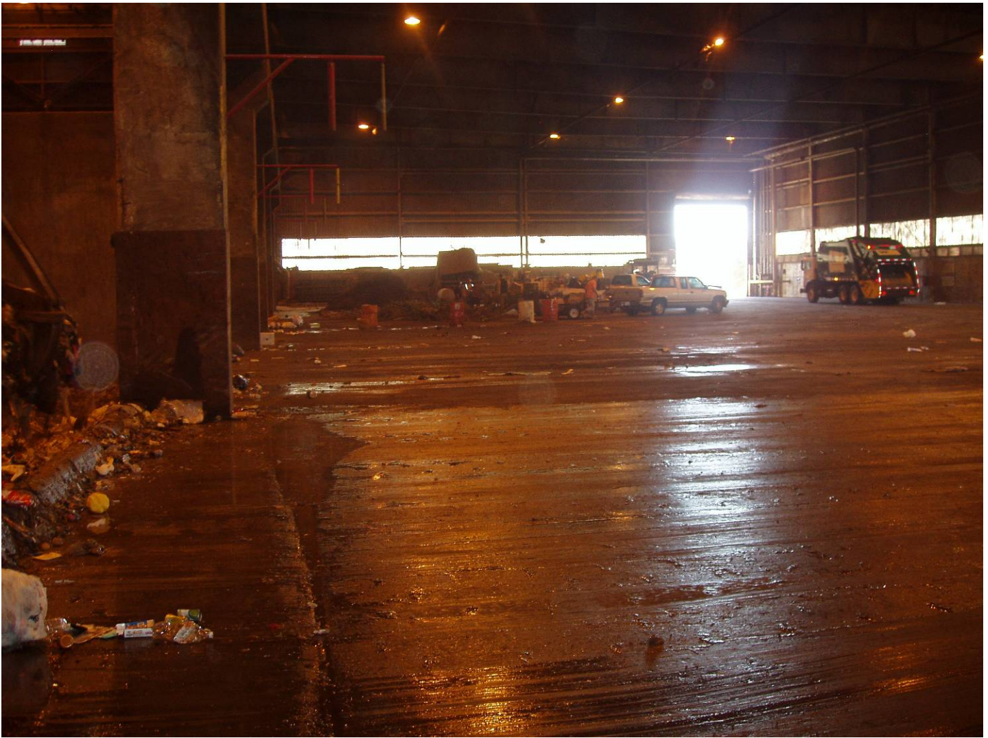
Photo ID: 1010056_Photo_01_20_2012-2; Time: 01/20/2012, Approx. 11:00 A.M. Building for trash drop-off at the Pasco County Resource Recovery Facility. The trash pit is shown on the right of the photograph.
