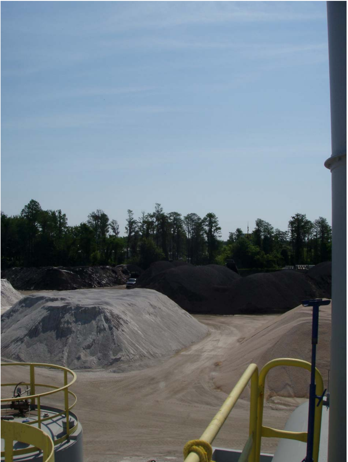
Photo ID No: 1010027_Photo_04_10_2012-020 Time: Approx. 11:00 AM Storage piles for raw materials and broken pieces of asphalt and crushed pieces of asphalt. The camera is facing approx. E.
