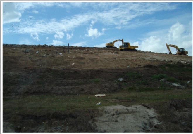
Photo 17: W view of active landfill cell.
