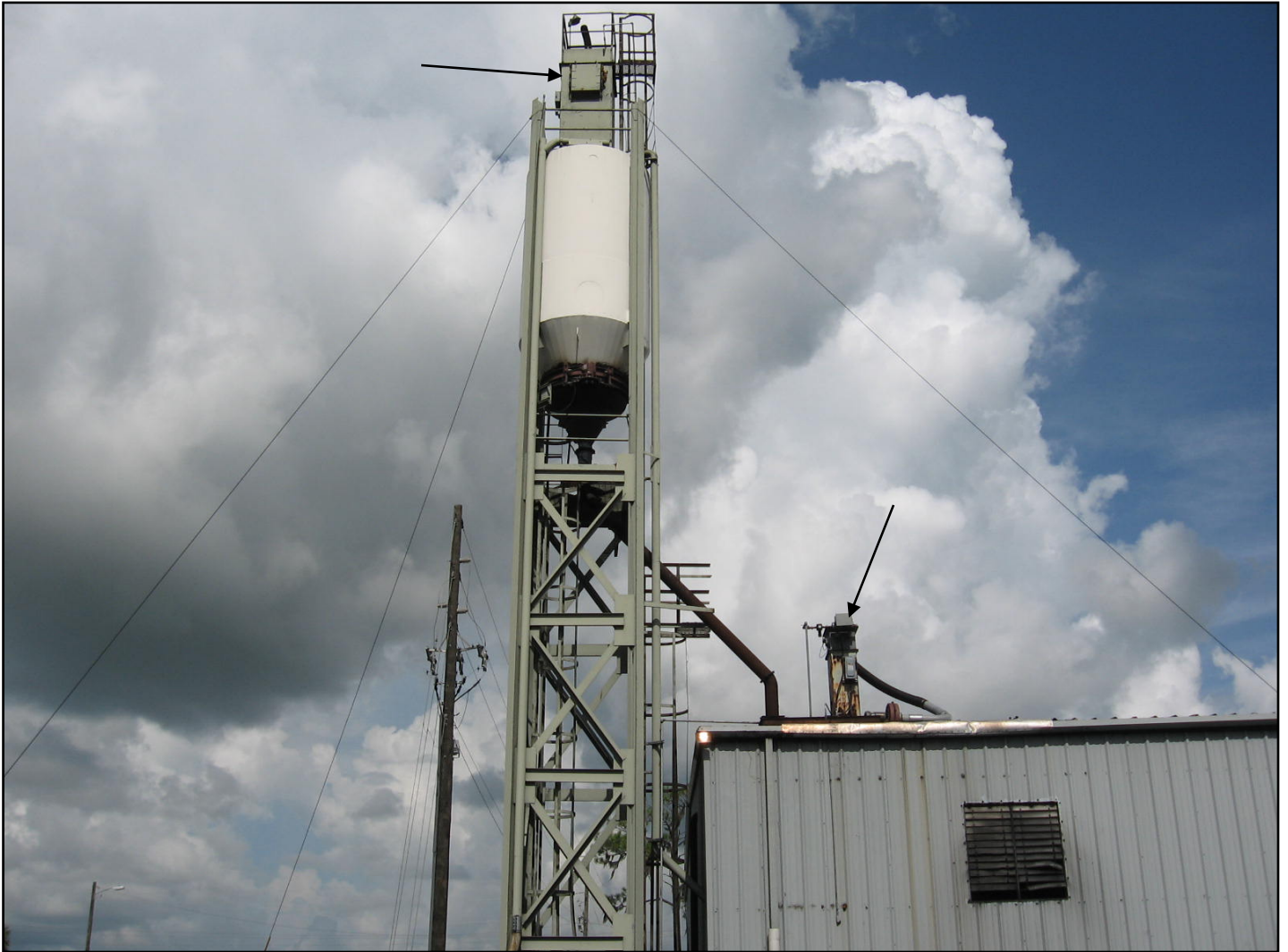
Photo ID No. / Date / Time: IMG_1334 / 07-12-11 / 1037 Flex-Kleen and Mahle baghouses
