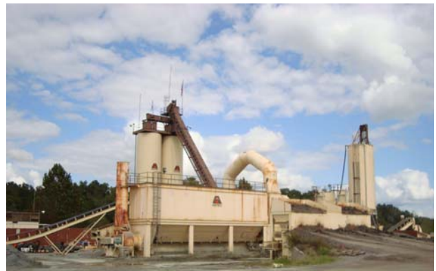
The asphalt plant.
