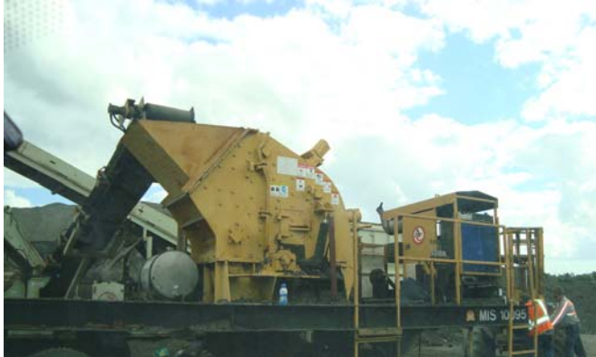
Crusher unit and engine located to the right.
