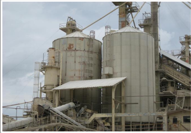
Photo 5: Tanks #7 and #8 containing product.
