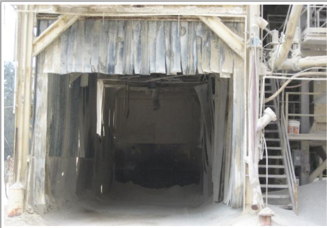
Photo 7: Front view of the load out area.
