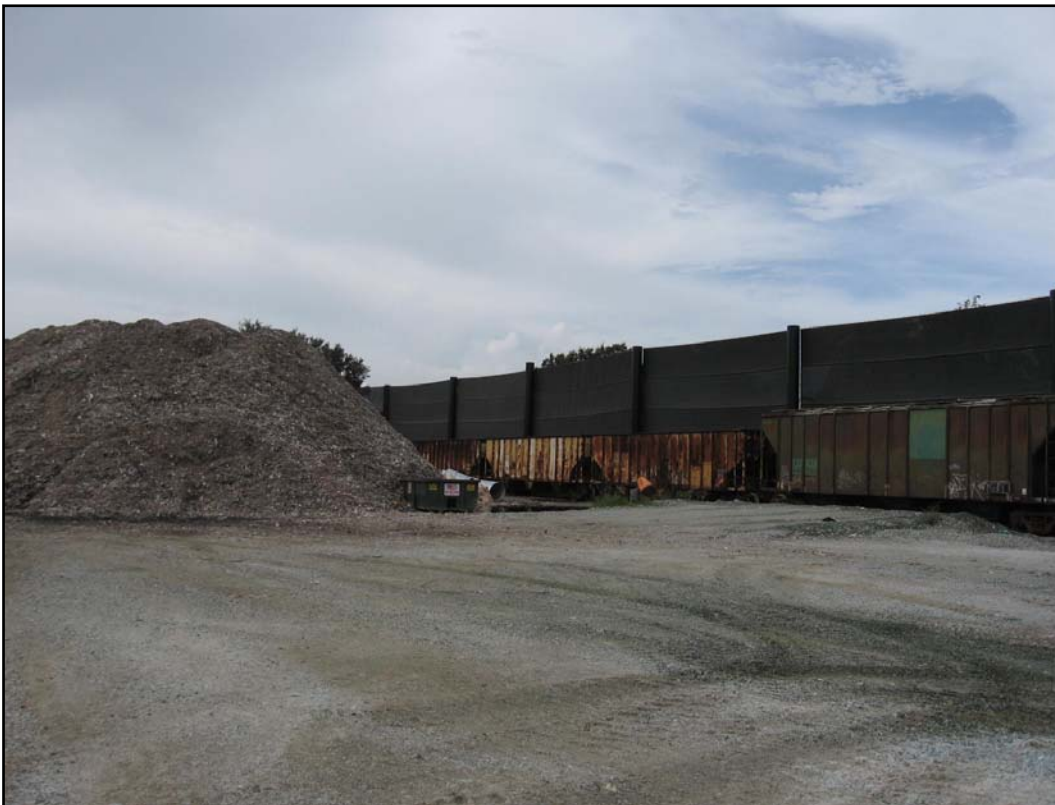
Photo ID No. / Date / Time: IMG_1447 / 08-15-12 / 0949 Recently installed windscreen
