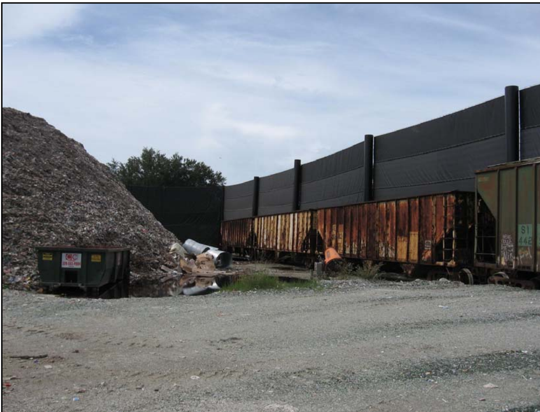
Photo ID No. / Date / Time: IMG_1453 / 08-15-12 / 1057 Recently installed windscreen (right) and waste pile (left)
