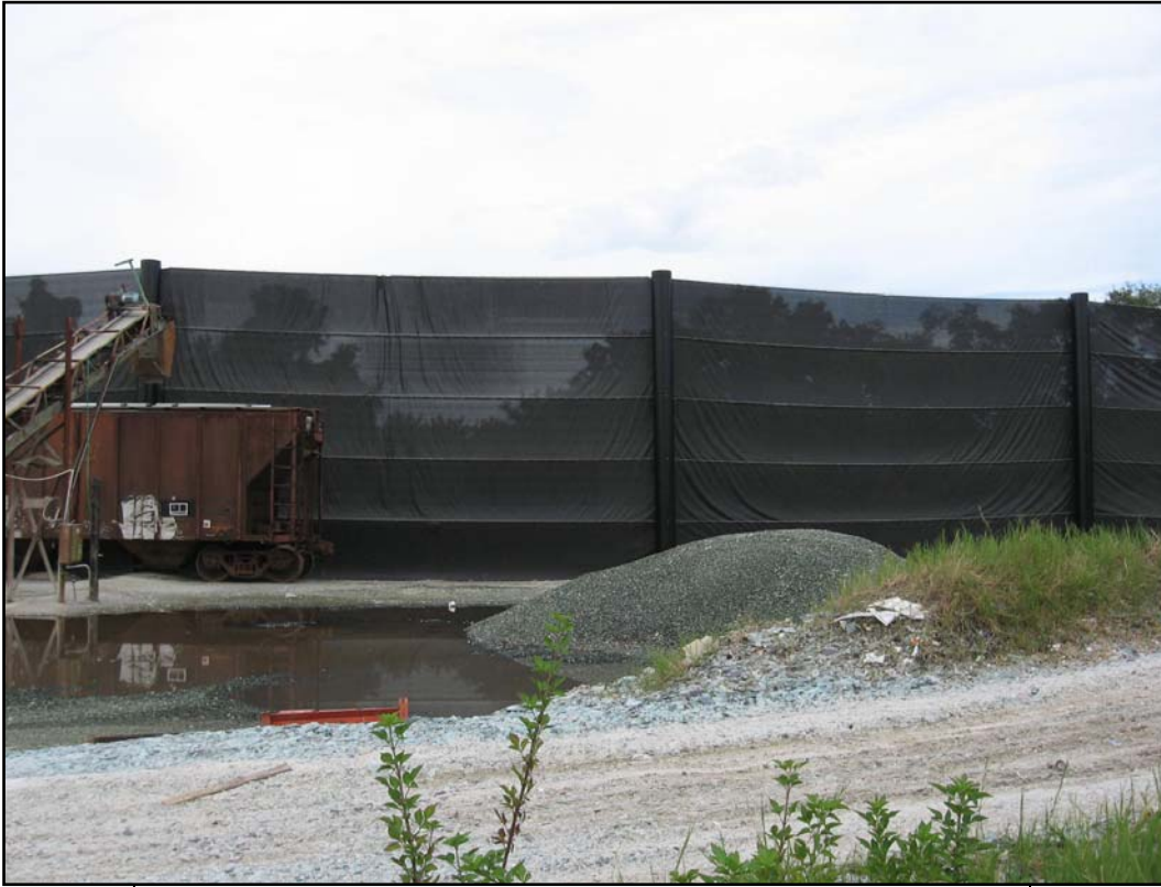
Photo ID No. / Date / Time: IMG_1446 / 08-15-12 / 0949 Recently installed windscreen
