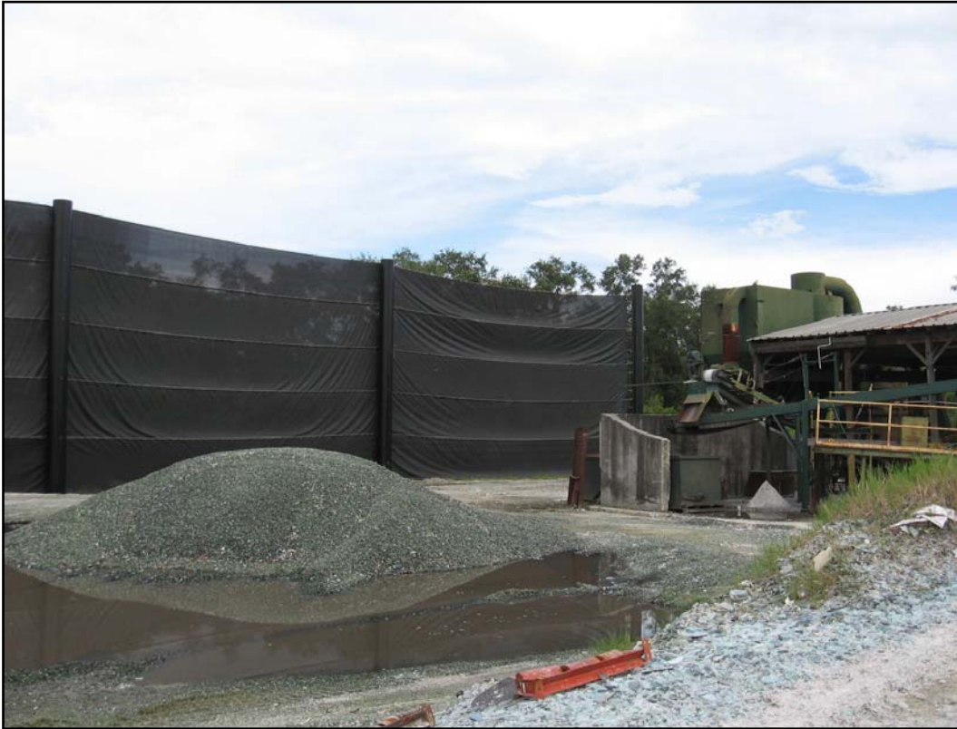
Photo ID No. / Date / Time: IMG_1448 / 08-15-12 / 0950 Recently installed windscreen
