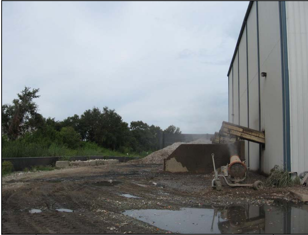
Photo ID No. / Date / Time: IMG_1450 / 08-15-12 / 1010 South side of Line No. 1 building
