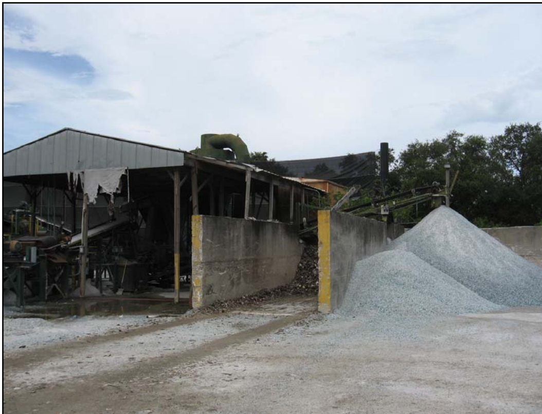
Photo ID No. / Date / Time: IMG_1445 / 08-15-12 / 0948 Old glass processing line (Line No. 2)
