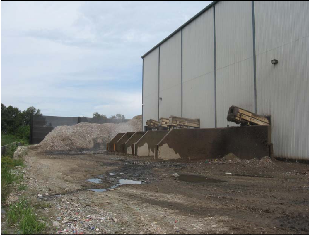
Photo ID No. / Date / Time: IMG_1452 / 08-15-12 / 1013 South side of Line No. 1 building
