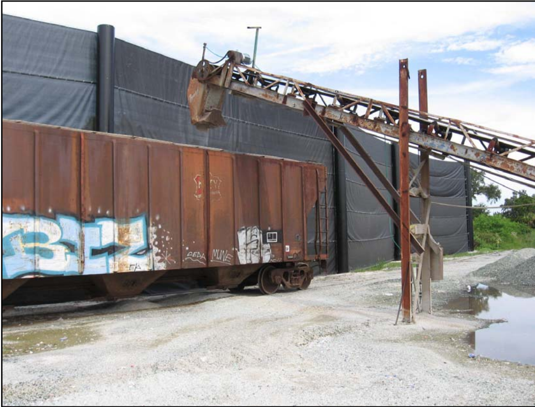
Photo ID No. / Date / Time: IMG_1454 / 08-15-12 / 1057 Recently installed windscreen
