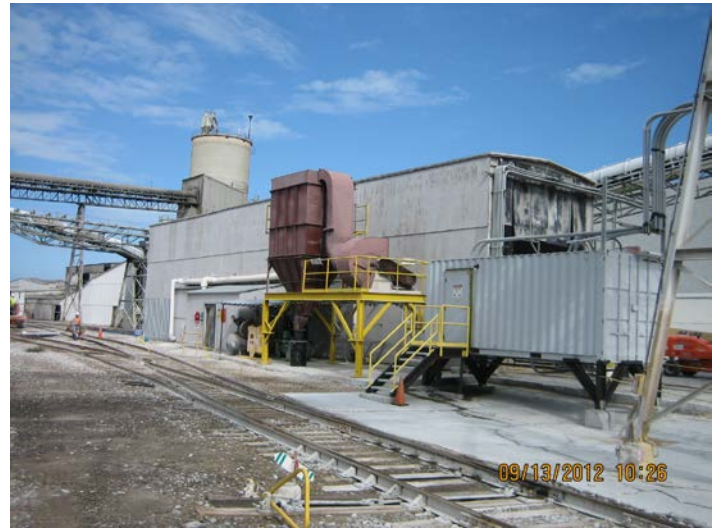
Photo ID No: IMG_430—Emission Unit No. 001 and Railcar Unloading Building
