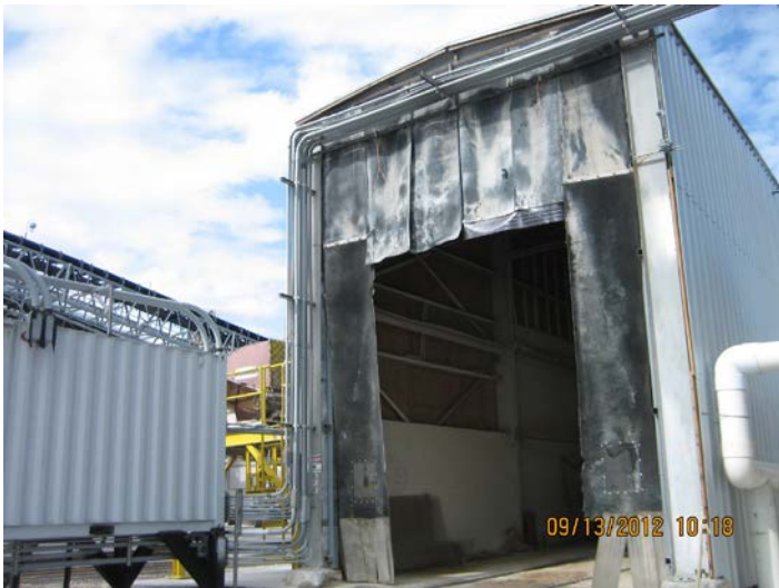
Photo ID No: IMG_429—Railcar Unloading Building
