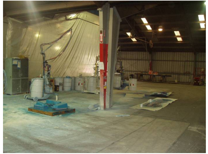
Photo ID No: Photo_0530363_02_23_2012-15 Time – Approx. 11:15 AM Location for storing and using gelcoat in barrels. The camera is facing approx. NE.
